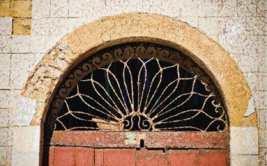
Bandeira vazada. Transom light.
