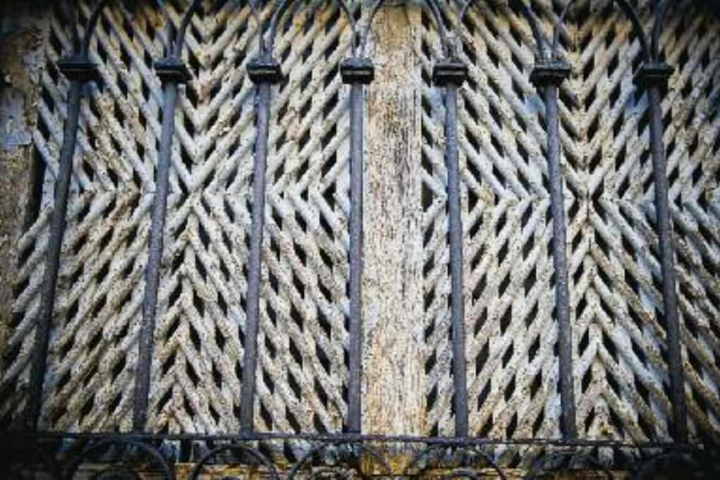
Screens of trellised wood placed on balconies to avoid exposing the interior of dwellings. Sol Street, 311.
