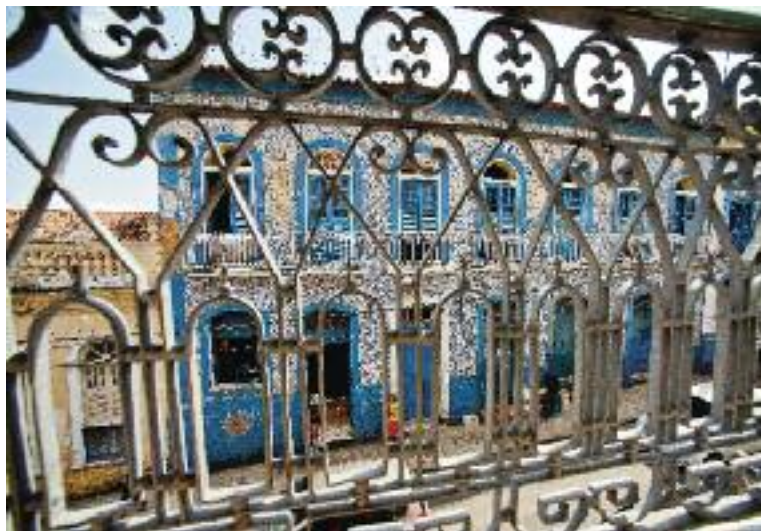
Gradis de balcões. Balcony railings.
