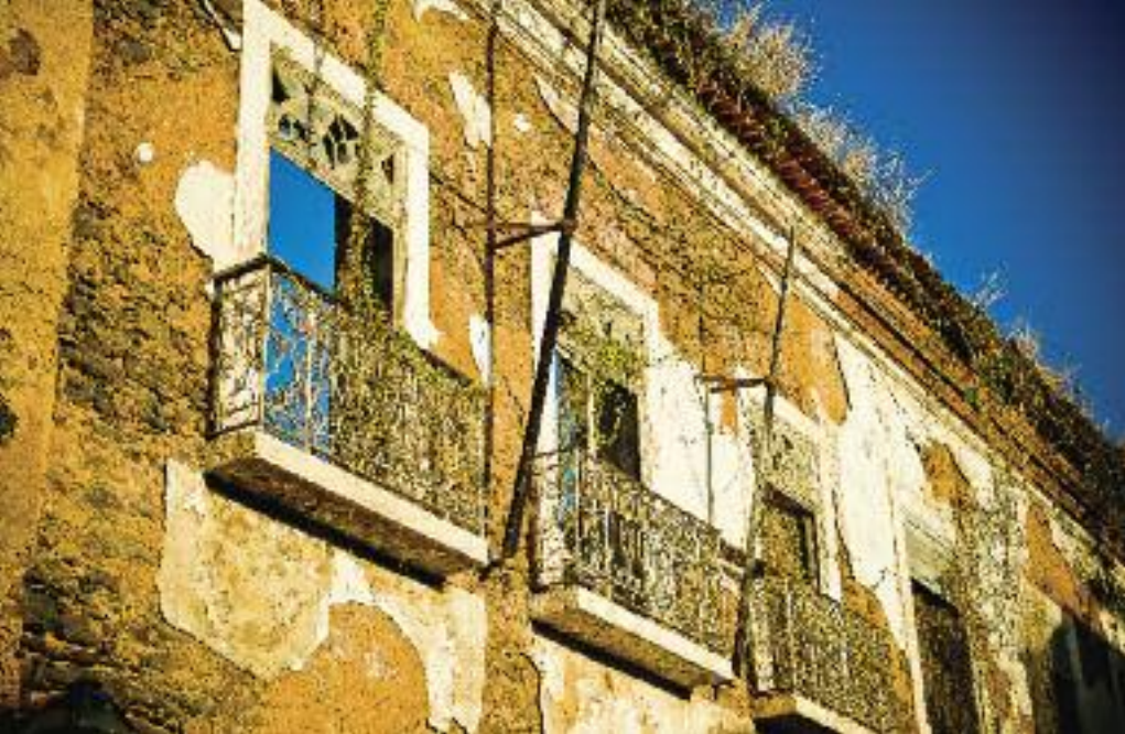
Alvenaria de pedra e cal. Stone and lime masonry.
